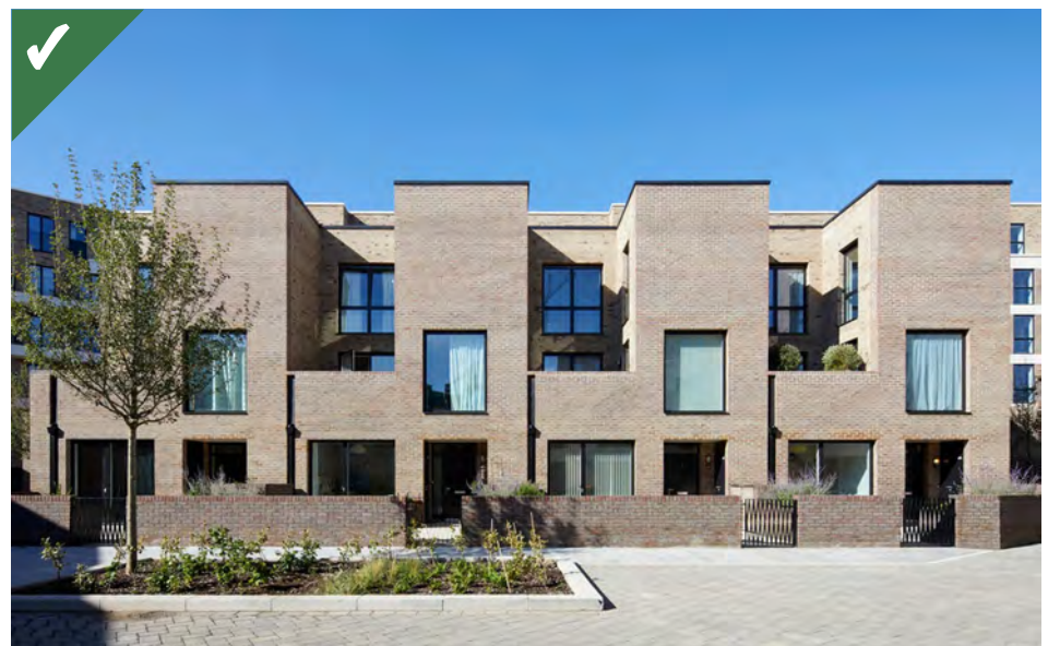
Figure 2.24c: Generously sized openings help to break up the mass of new terraced homes designed by Haworth Tompkins. Their position adds rhythm to the elevation. (Photo: Jack Hobhouse)
