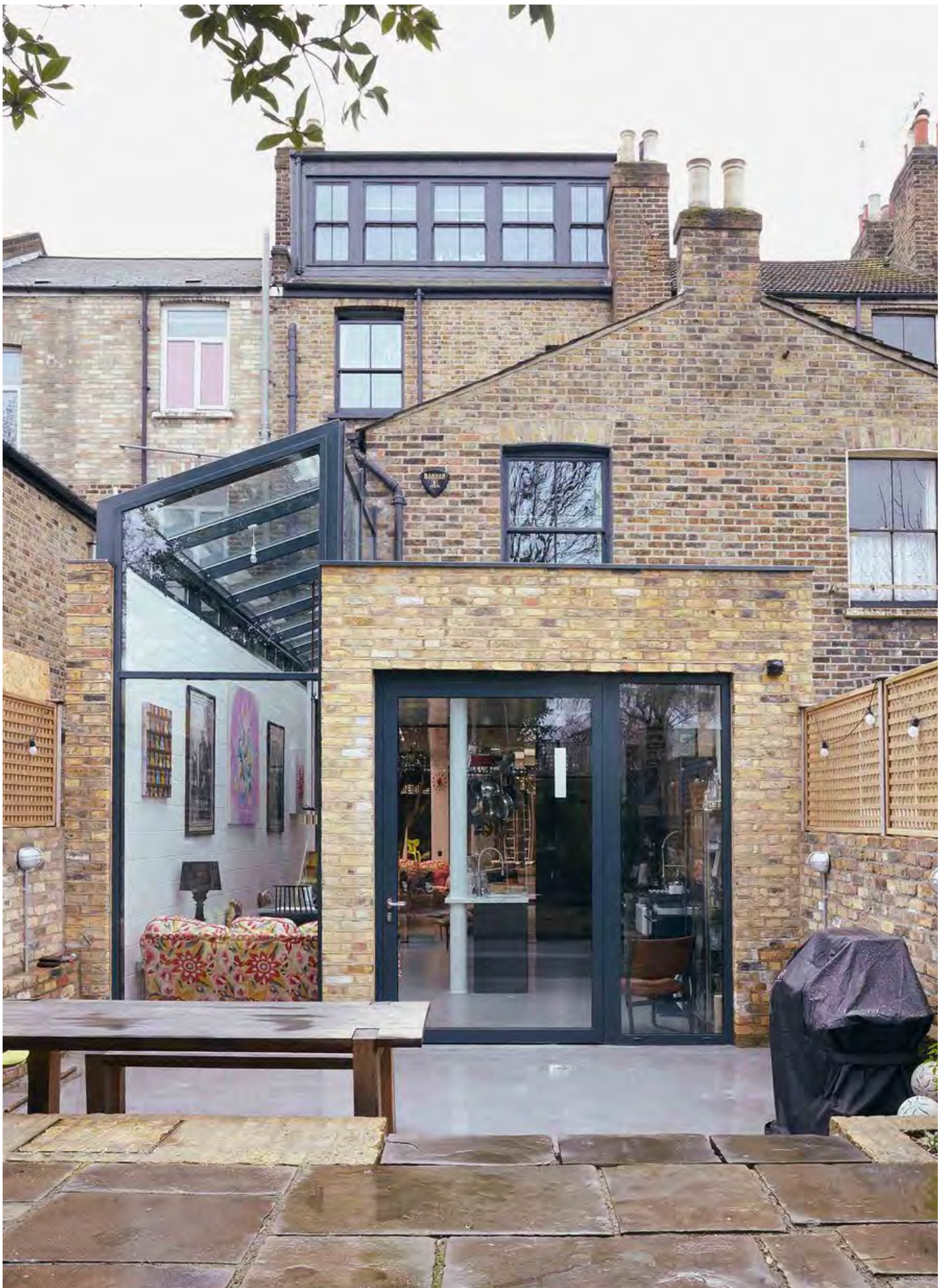
Figure 4.5c: A series of extensions designed by fourth_space that appear supplementary to the original house by clearly responding to its existing form and materials.
