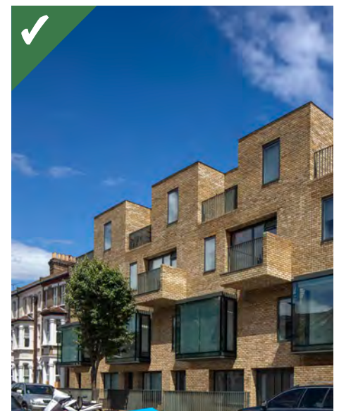
Figure 2.26c: A combination of recessed and cantilevered balconies are provided in this development designed by Peter Barber Architects that provide rhythm to the scheme and allow it to successfully sit alongside a traditional terrace. (Photo: Morley von Sternberg)
