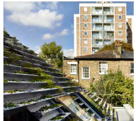
Figure 2.36c: Stepped roof with planters designed by Hayhurst & Co.
