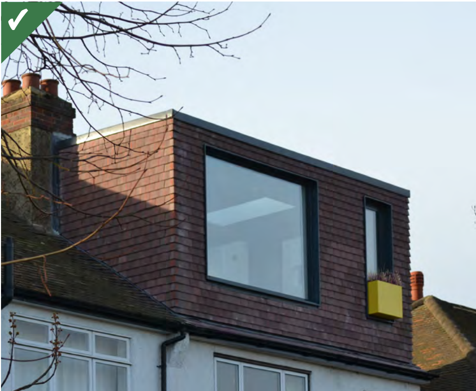
Figure 4.21c: A good example of a box dormer on the rear of a terrace house successfully designed by Selencky Parsons to integrate into the existing dwelling; the dormer replicates existing roof tiles, conceals rainwater pipes and aligns the glazing with the windows below. The dormer provides a generous amount of glazing, avoiding an overbearing appearance and benefiting the internal spaces.
