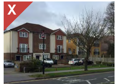
Figure 2.17d: A development which appears wide and squat as a result of poorly considered proportions and fenestration
