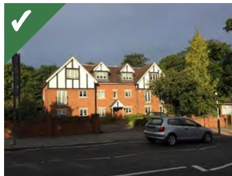
Figure 2.17c: A wide development which has successfully dealt with its width through proportions and fenestration
