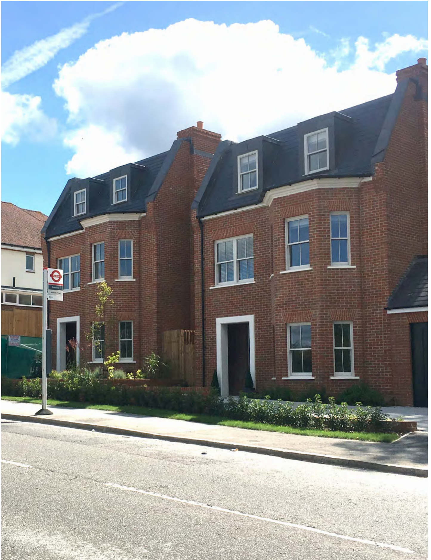
Figure 2.19a: A street facing development of family homes on Purley Downs Road. The development provides accommodation within a mansard roof.
