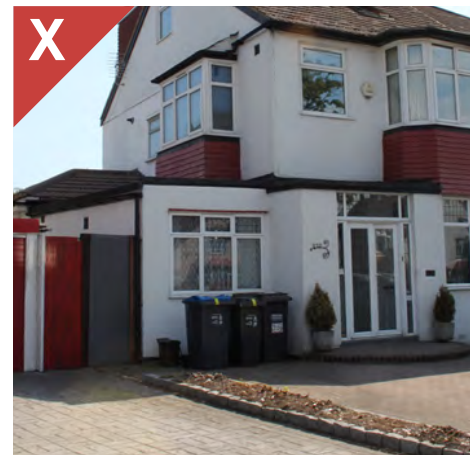
Figure 4.12b: A poorly designed single storey side extension that fails to respond to the original dwelling. It has an awkward combination of roof forms and the appearance is further exacerbated by the porch extension, which hasn't been combined with the side extension.
