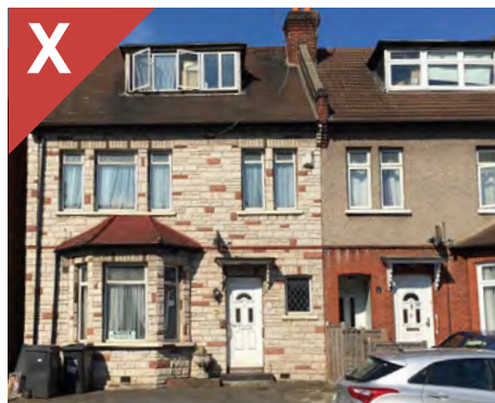
Figure 4.26d: An example of inappropriate cladding to a house that hinders the appearance of the street.
