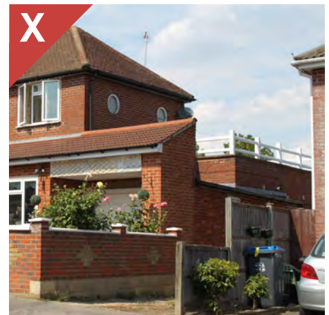
Figure 4.15b: A side and front extension with a series of different roof forms results in a poorly considered composition that has a negative impact on the streetscene.
