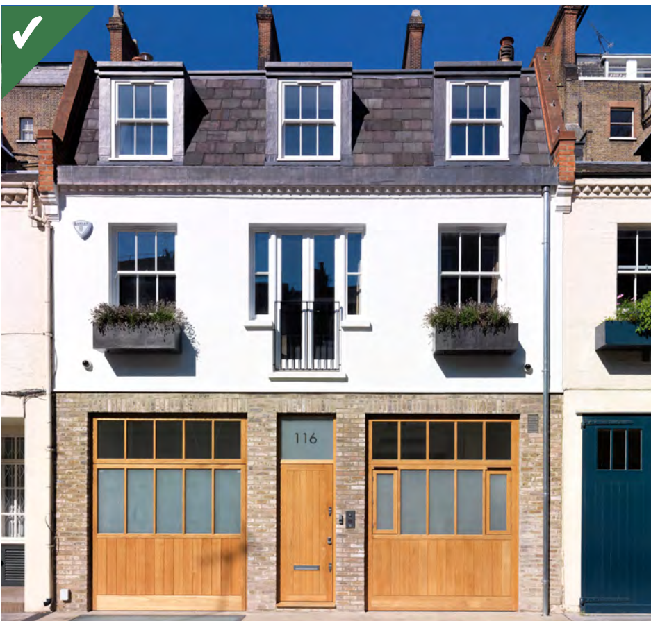
Figure 4.21d: The addition of 3 dormers by Threefold Architects that have been sympathetically designed to the existing building and respond to the positioning of the windows below.
