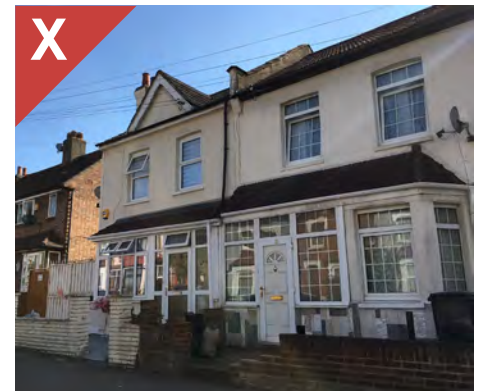
Figure 4.14b: A poor example of two porches that have been built up to and over original bay windows. The design fails to respond to the historic pattern of development and materials are low quality.
