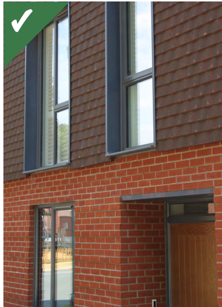
Figure 4.25a: A wall with different depths of window and door reveals. Deeper reveals add emphasis and solidity to the appearance of a house.
