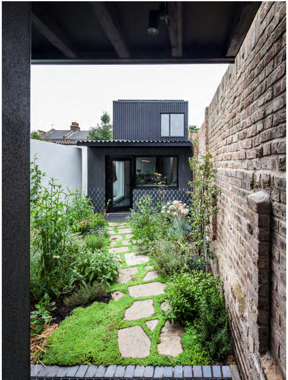
Figure 2.18a: A rear-garden house designed by Dallas–Pierce–Quintero that builds along the boundary wall. (Photo: David Butler)
