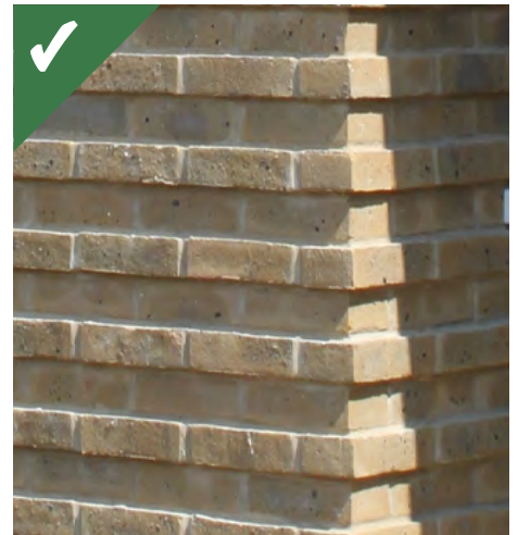
Figure 4.27e: Stepped courses of brickwork.
