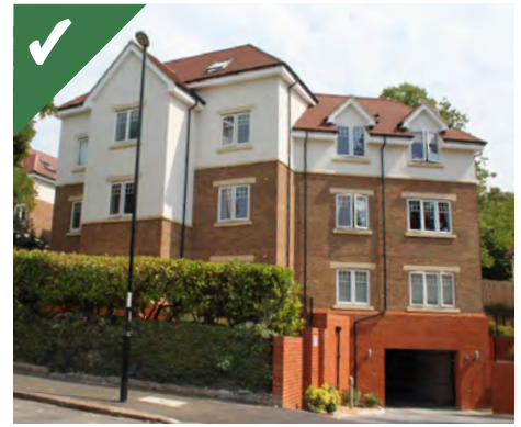
Figure 2.30b: The use of a basement for parking allows the front garden to remain predominantly planted.
