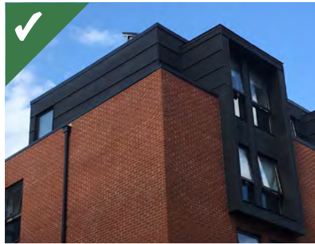
Figure 2.19b: Flat roof forms are acceptable. Set-back top floors with a change in material can be used to add interest and break down the mass.
