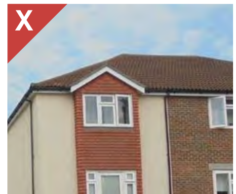
Figure 2.19f: Pitch of roof appears too shallow in relation to mass of building.
