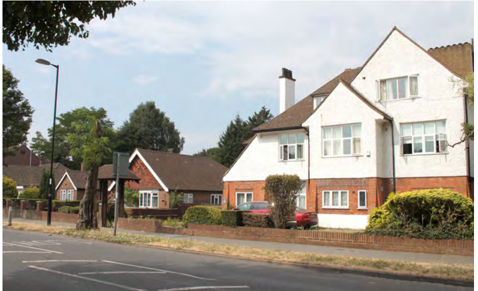
Figure 2.10a: A development of 3 storeys containing flats sits next to a bungalow and does not appear overbearing.
